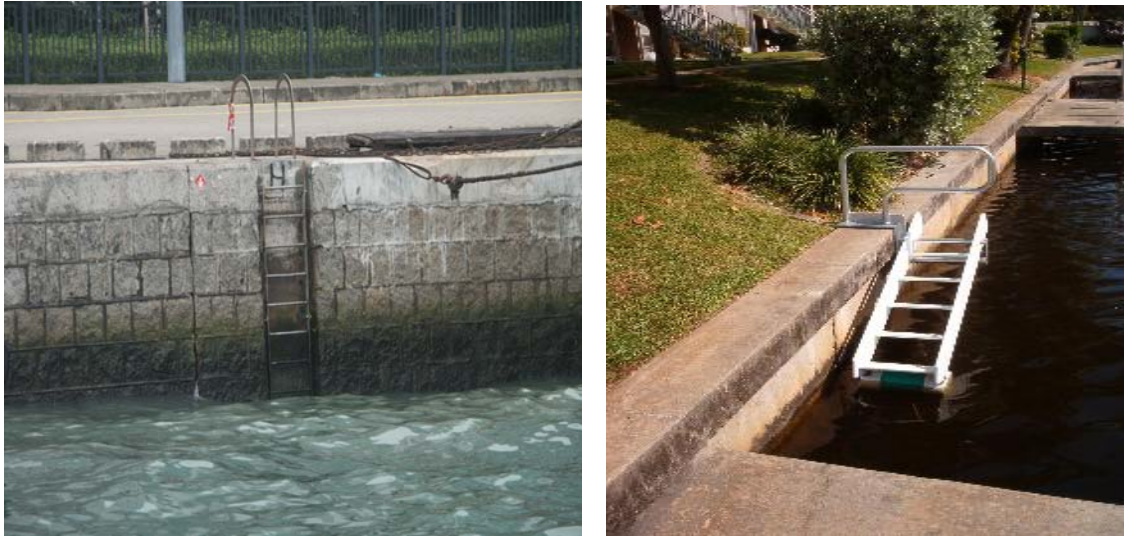
Photo 4 – Pier Ladders 圖4 – 碼頭梯
