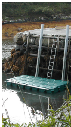
Photo 9 – Airfloat Pontoons
