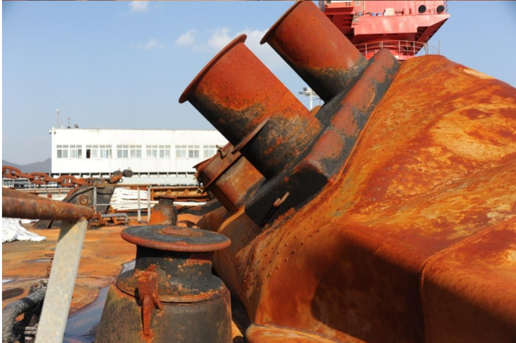
Fore-castle deck bending backwards
