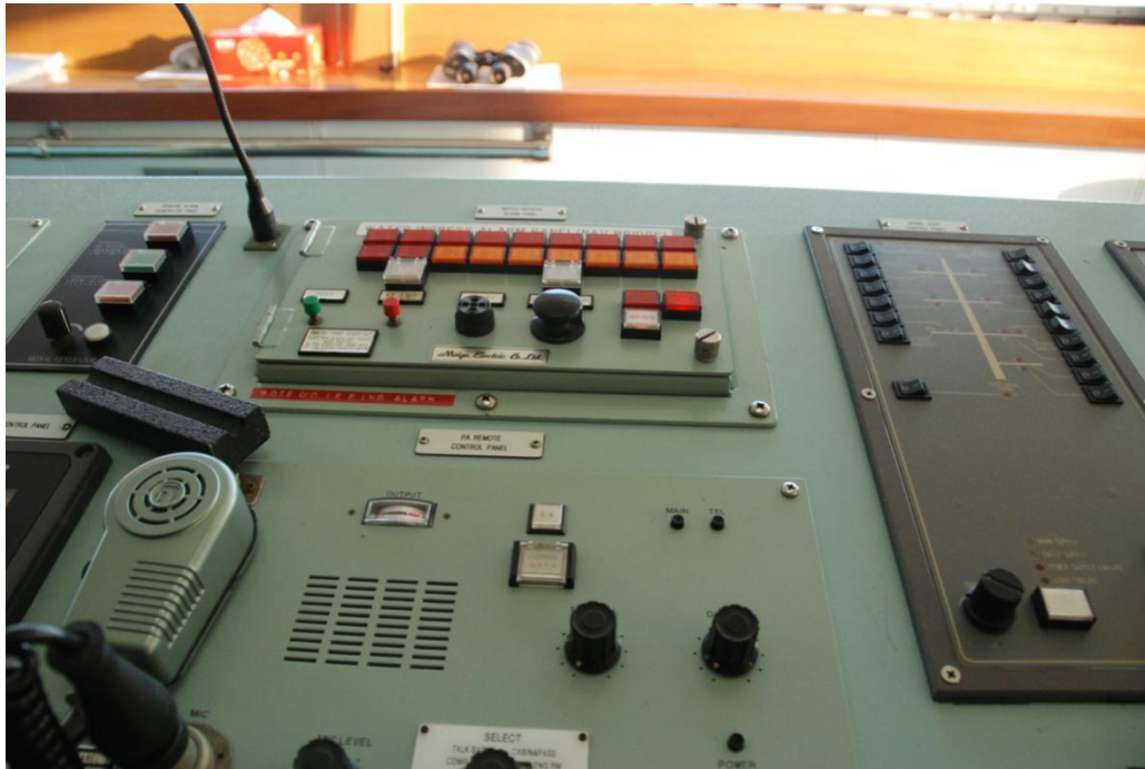
Public Adress System
