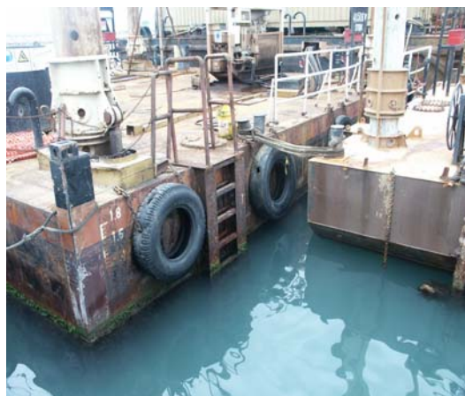
Photo 9 –Fixed ladders on lighters
