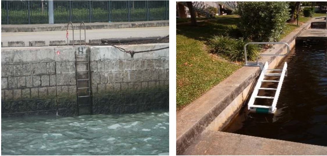
Photo 4 – Pier Ladders 圖4 – 碼頭梯
