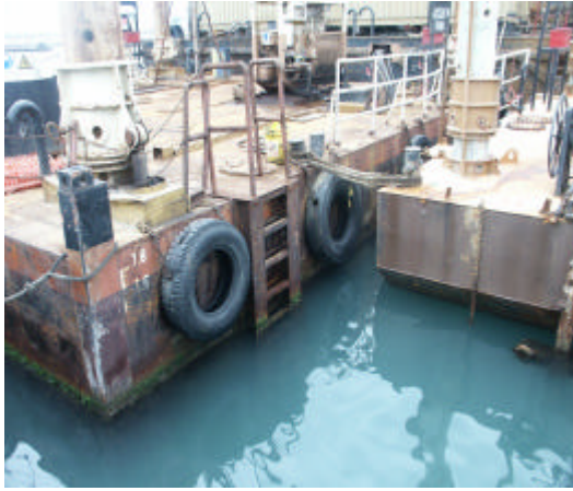
Photo 9 –Fixed ladders on lighters
