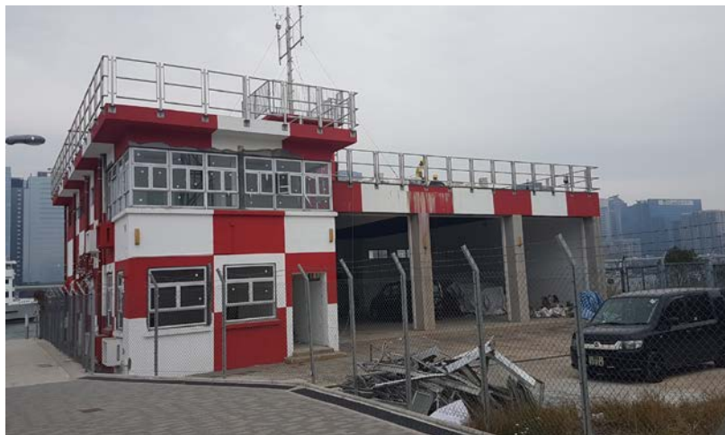
Photo of the Former Fire Station Building
