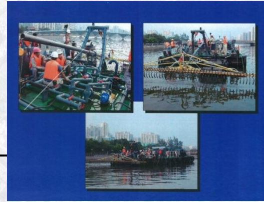
以生物除污法處理受污染海牀底泥 (啓德明渠進口道及觀塘避風塘) Treatment of Sediment by Bioremediation (KTAC and KTTS)
